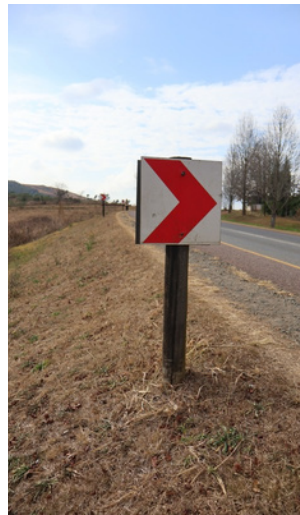
Road signs installed at Tweedie off-ramp (July 2025)
