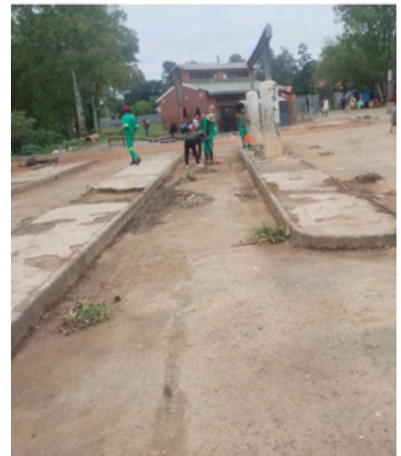
Pavements in Harvard, Bell, and Morling Streets repaired
